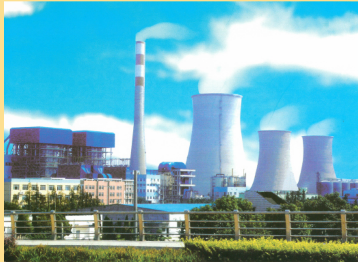
Boiler of Power Station
